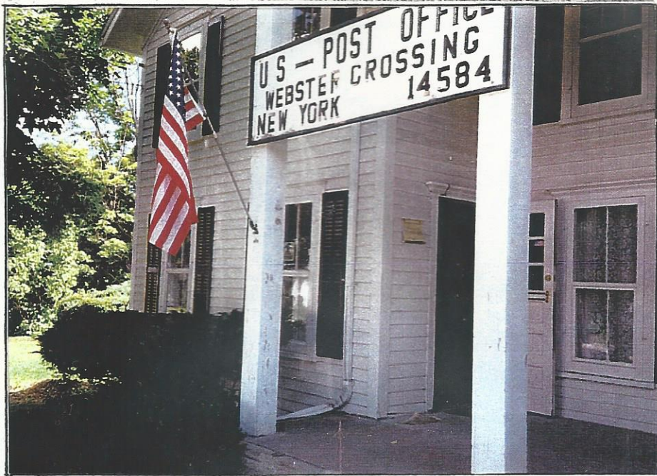
Last home of the Webster Crossing U.S. Post Office 7273 Route 15, Webster Crossing, N. Y., 14584
