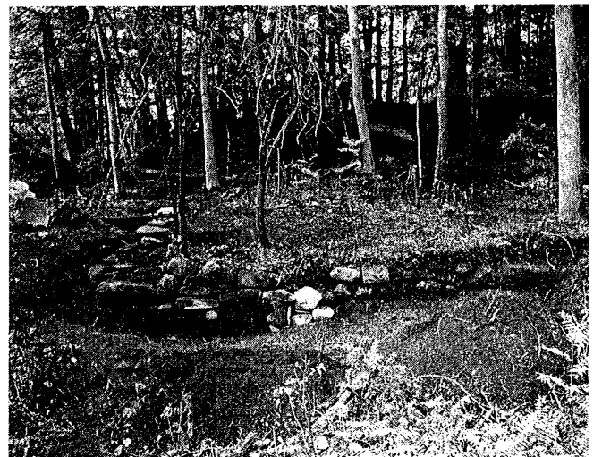
Figure 19. Grove Mather House foundation, view looking north.
